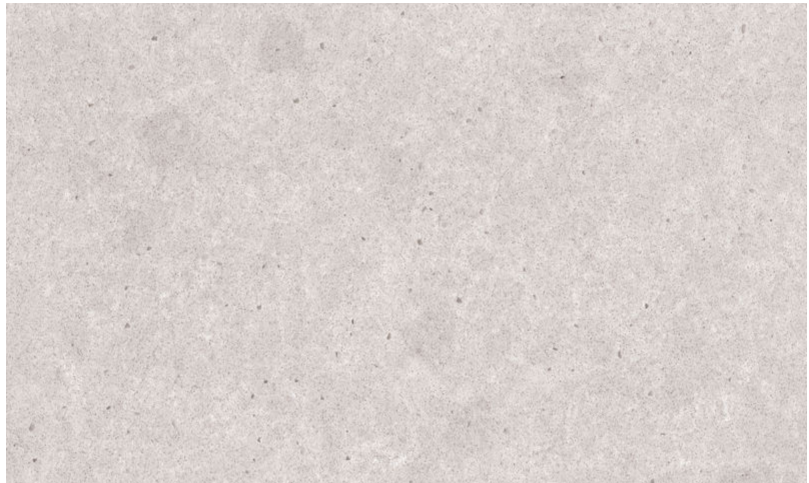
FULL SLAB VIEW
